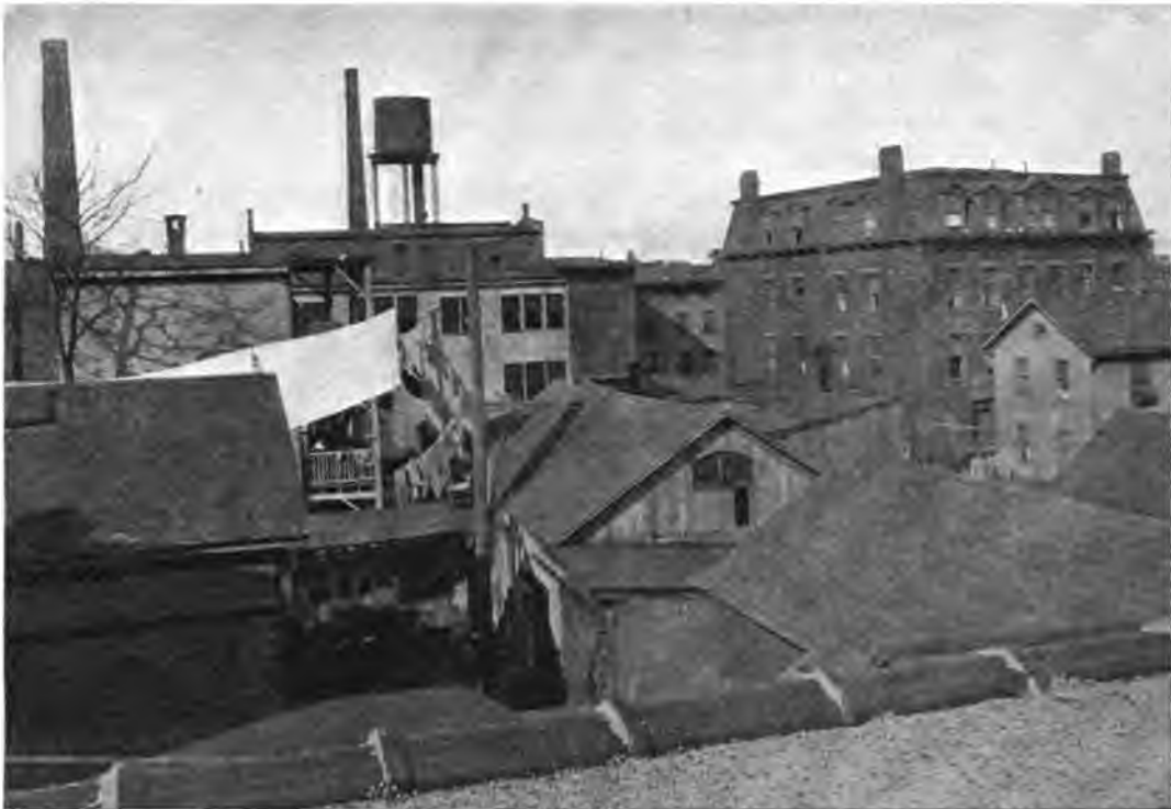
Interior Reilley Street block
